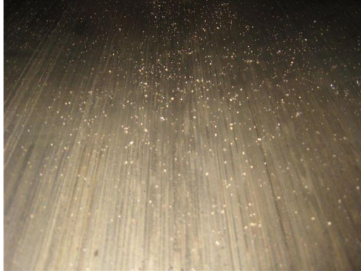
Figure 3: Damage to running surface
